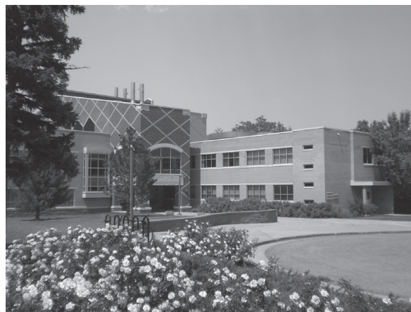
Fig.1 Building of ASPPRC.
