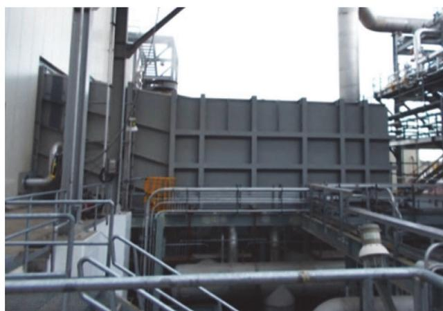
Fig.12 The externals of direct contact condenser. (Online version in color.)
